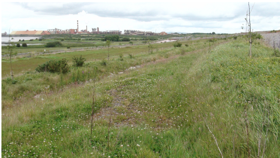
Figure 12. Side slope rehabilitation.
